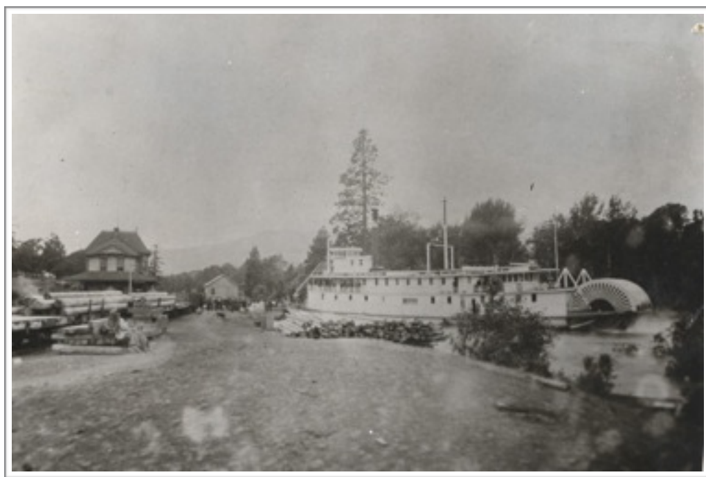
Steamer "Regulator" at Rail Depot, Flood of 1894
