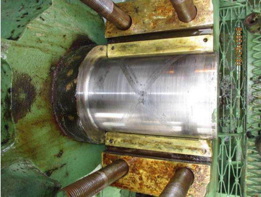
Figure 16: Typical bottom half of trunnion bearing journal after cleaning.
