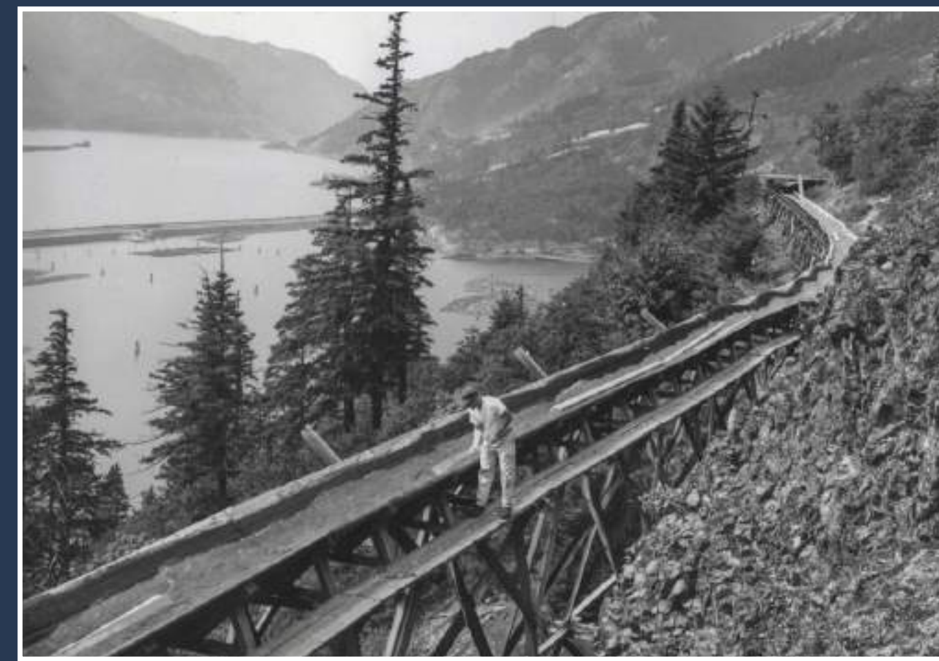
The Broughton Flume (sections of which are still visible) brought logs from Willard, WA to the Broughton Mill on the Columbia 5 miles west of here.
