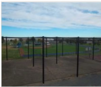
UAV/Drone Enclosure – Big Bend Community College, WA
