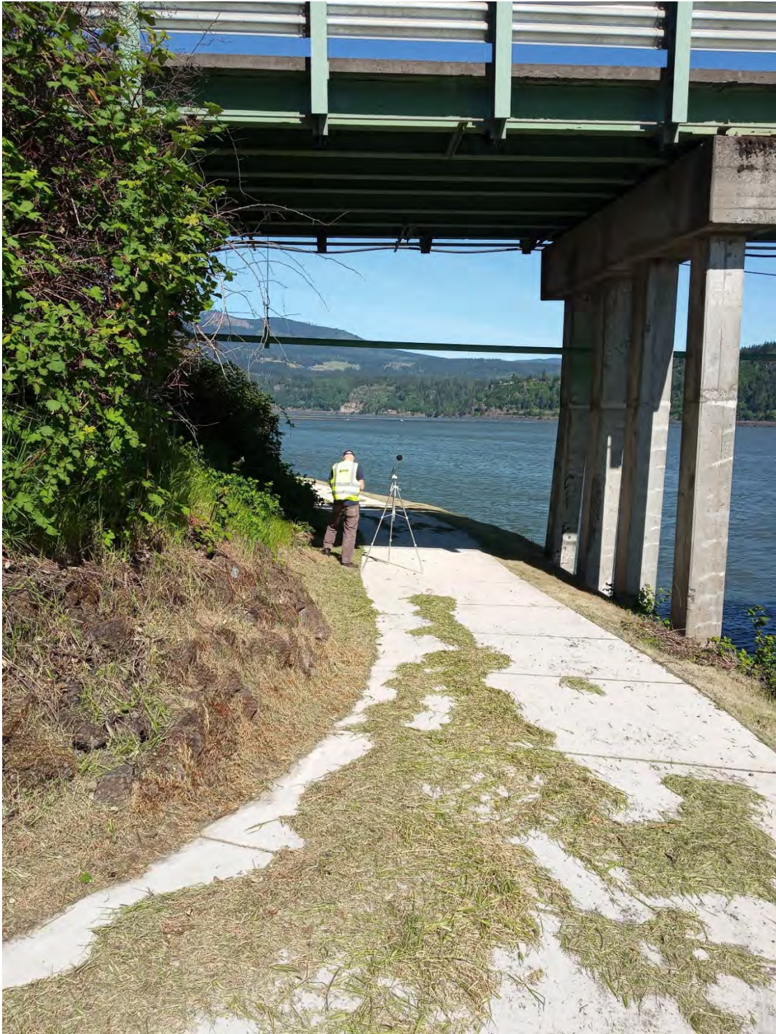
Figure 6: Waterfront Trail Crossing Under Hood River Bridge Source: WSP USA, Inc.
