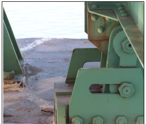
Figure 3 2008 Photo at Pier 3
