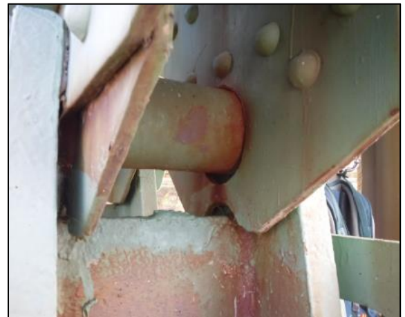
Figure 4 Torch-cut repair at Pier 19
