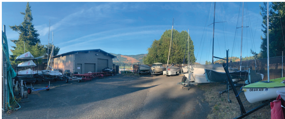
The fencing around the boat storage area for the Hood River Yacht Club will be expanded in 2022 and building improvements take place in 2025.
