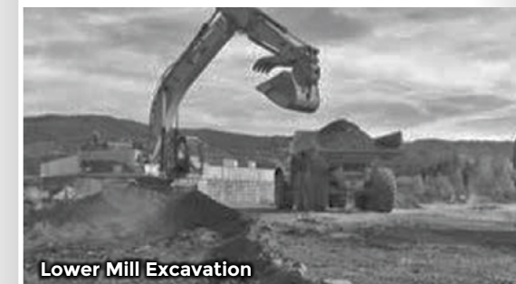
Lower Mill Excavation
