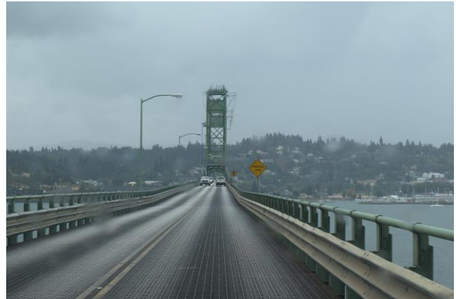
Hood River Bridge looking south
