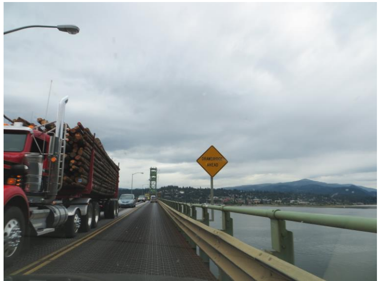
Narrow lane widths on grated steel bridge deck
