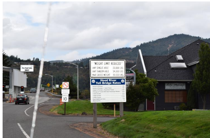
Toll and weight limit signs on northbound bridge approach
