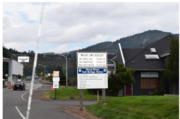
Too many signs at bridge approach
