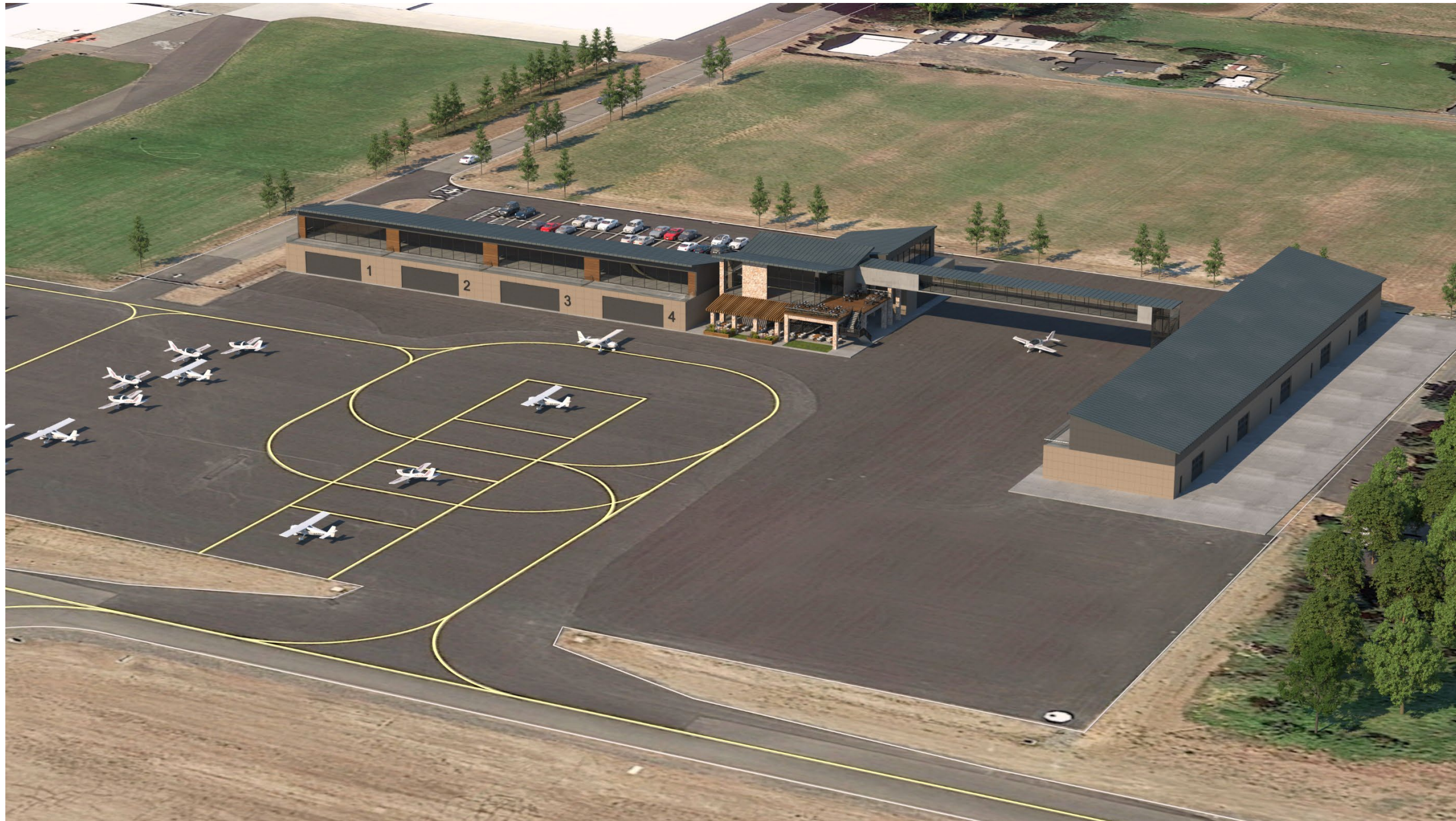
View to the northwest.
