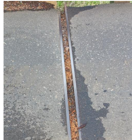
Figure 8. OR Abutment Joint
