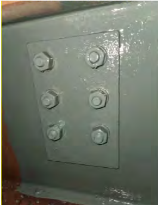
FLOORBEAM KNEE BRACE REPAIR- REPAIR #4
