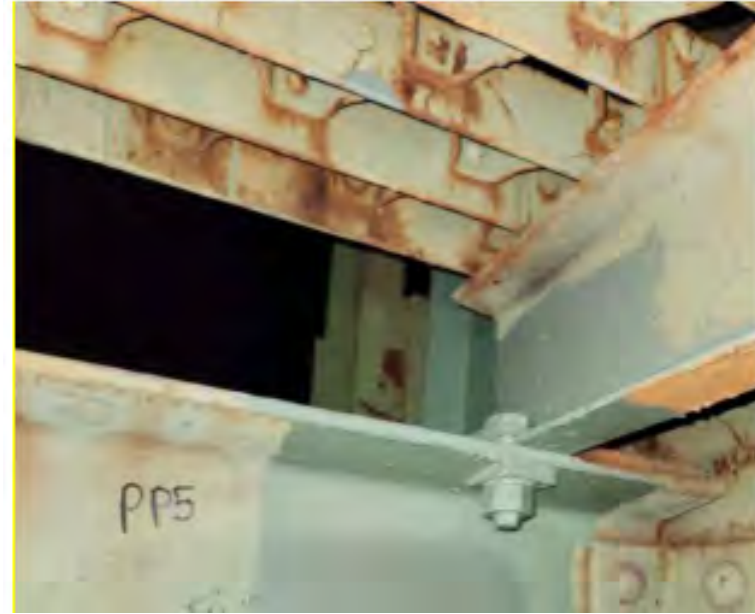
STRINGER TO SUB-STRINGER REPAIR #2
