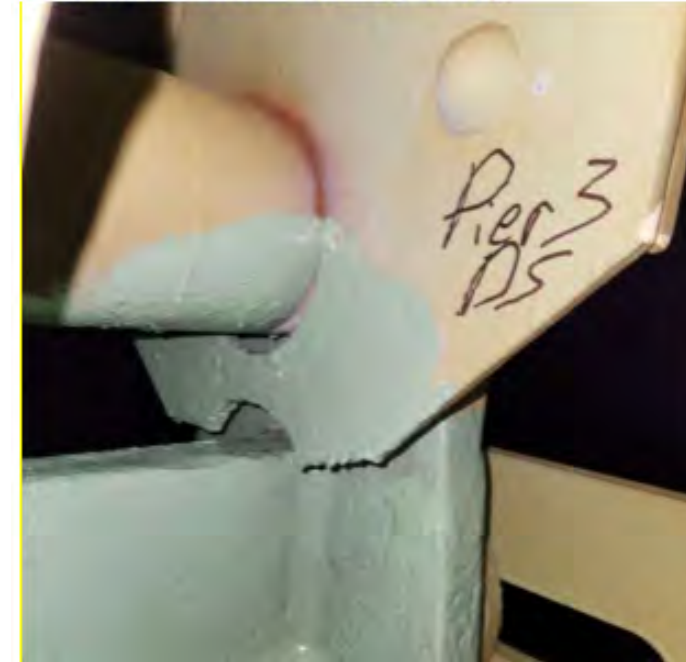
ROCKER BEARING MODIFICATIONS- REPAIR #6
