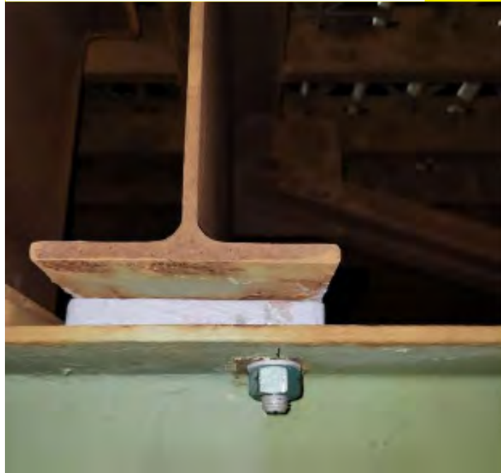
STRINGER TO FLOOR BEAM CONNECTION REPAIRS
