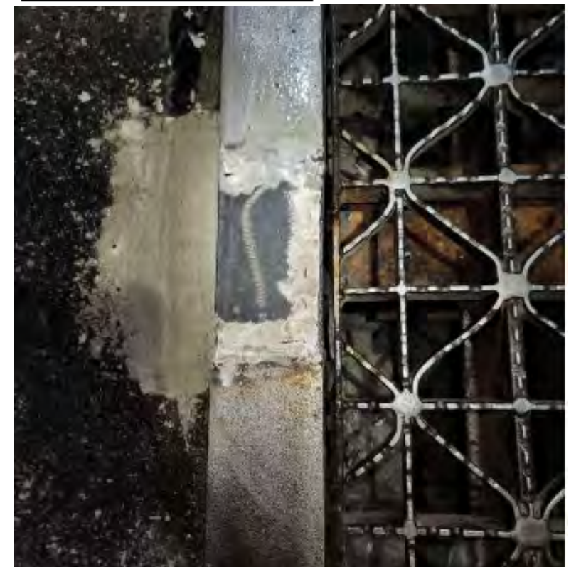
JOINT HEADER REPAIR
