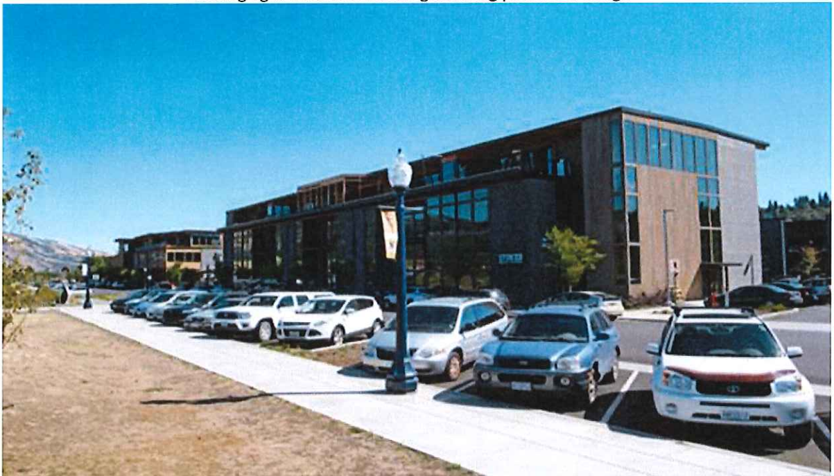
Existing light industrial building showing preferred design
