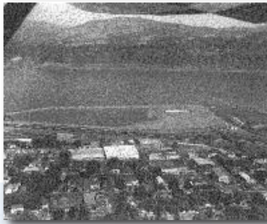
Waterfront development had a different meaning in 1964. This aerial photograph shows the fill in progress.
