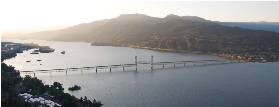
Figure 1-1. View of the Hood River-White Salmon Interstate Bridge
