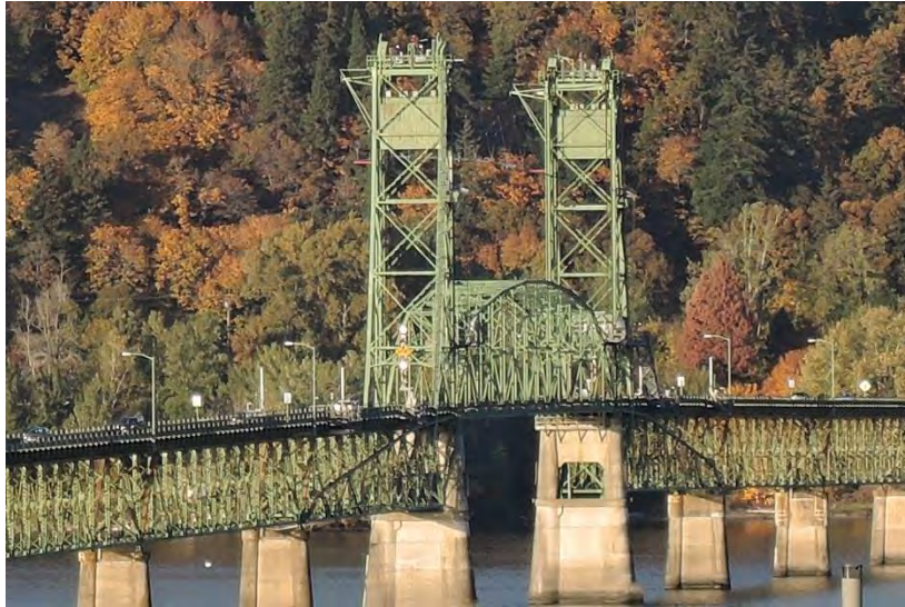
Figure 1. The Hood River Bridge is shown as viewed from the Oregon side of the river, looking North.
