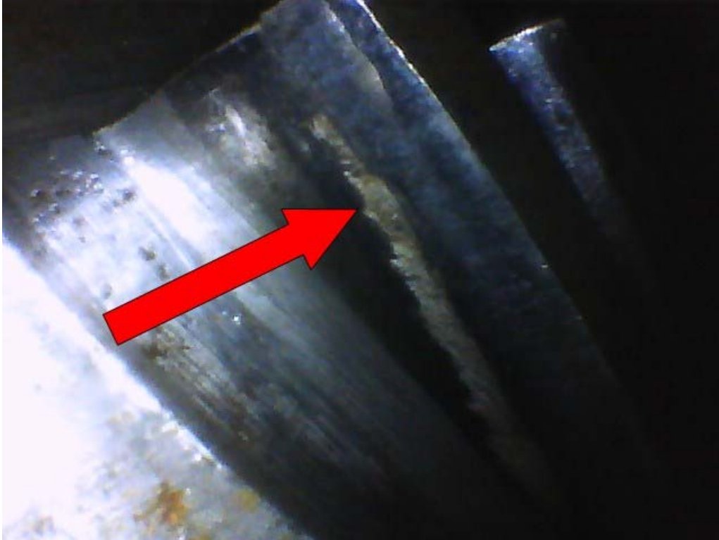
Photo 11 South Primary Reducer Gearing. View of west high speed pinion tooth. Destructive pitting extends across the width of the tooth at the pitch line.
