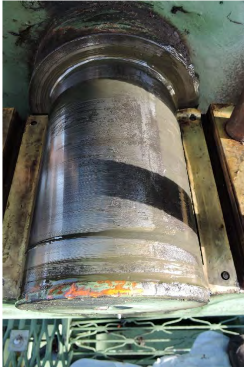
Figure 11. Corrosion pitting of the inboard journal of the southwest trunnion was indicative of contaminants within the bearing lubrication.
