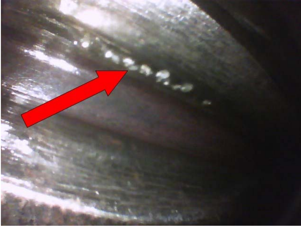
Photo 9 North Primary Reducer Gearing through Borescope. Note the pitting (arrow).
