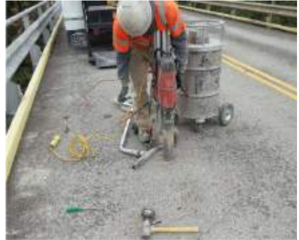
Figure 2. Core Drilling Apparatus
