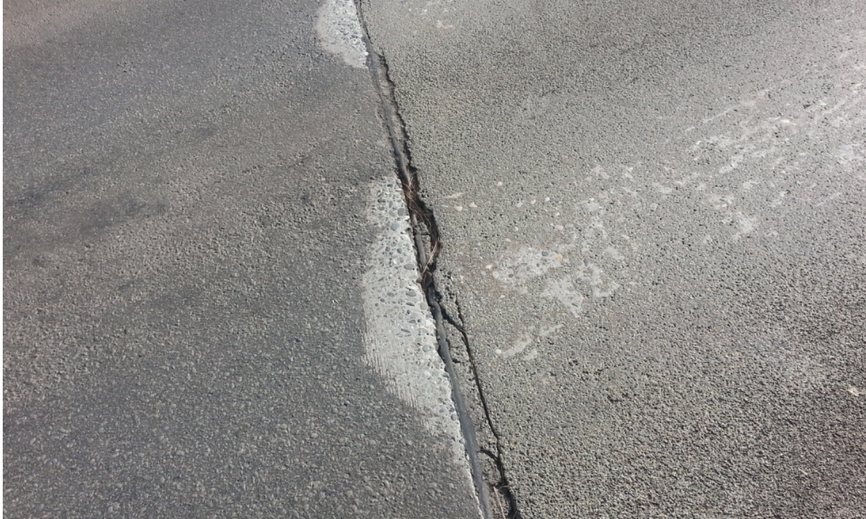
Joint at Washington Abutment (Bent 28).
