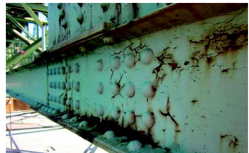
In 2011-2012, the Hood River Bridge underwent a major painting project as part of the Lower Chord Rehabilitation Project
