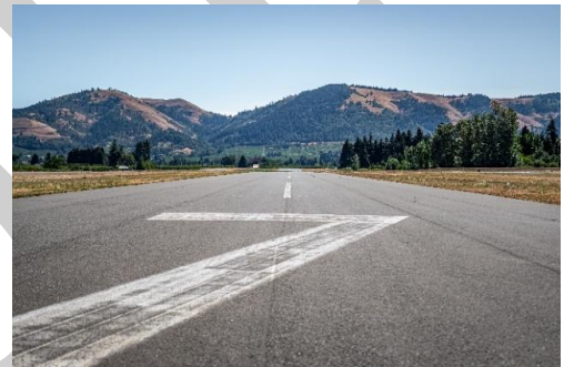
2012 Runway Shift work included relocating the runway, vacating a portion of Orchard Road and constructing a new road terminus
