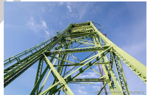
Major improvements during the 2000s extended the Bridge's operating life while replacement planning continued
