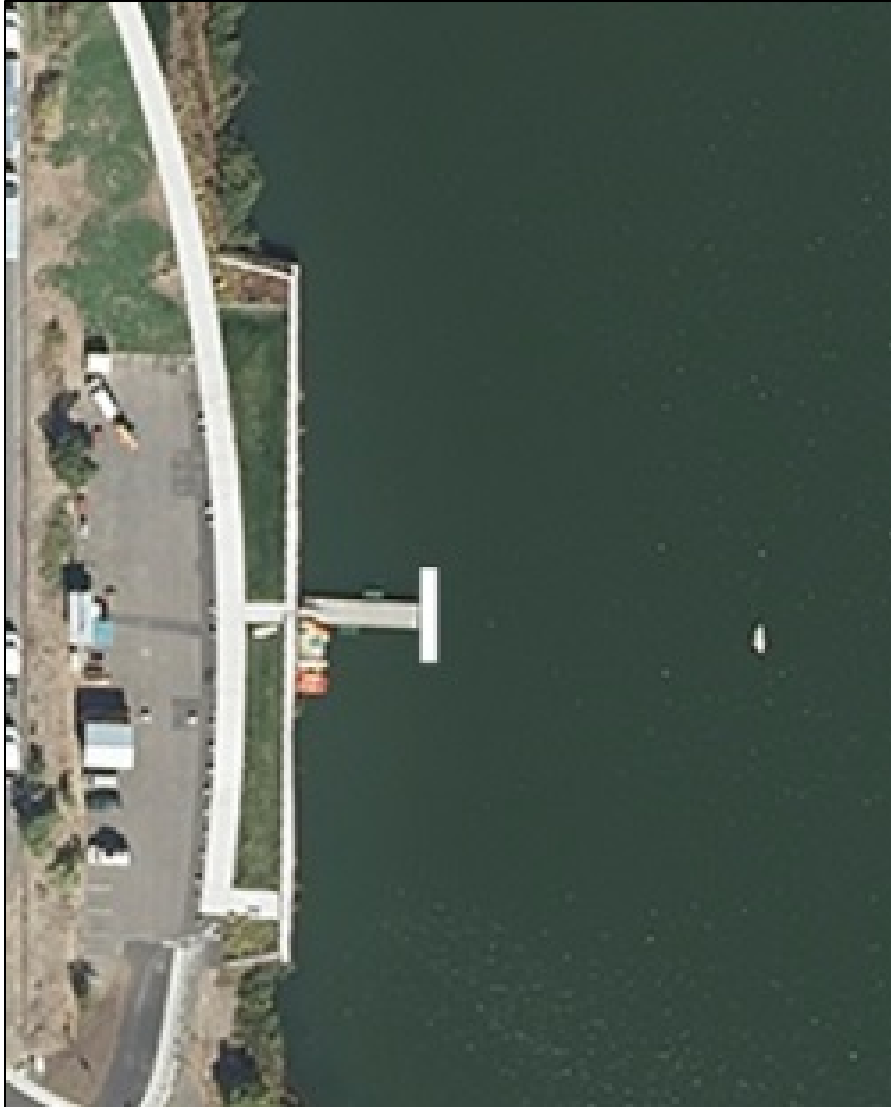
Aerial photo of the Nichols Basin, showing the existing dock with the proposed addition of a 30' concrete section.
