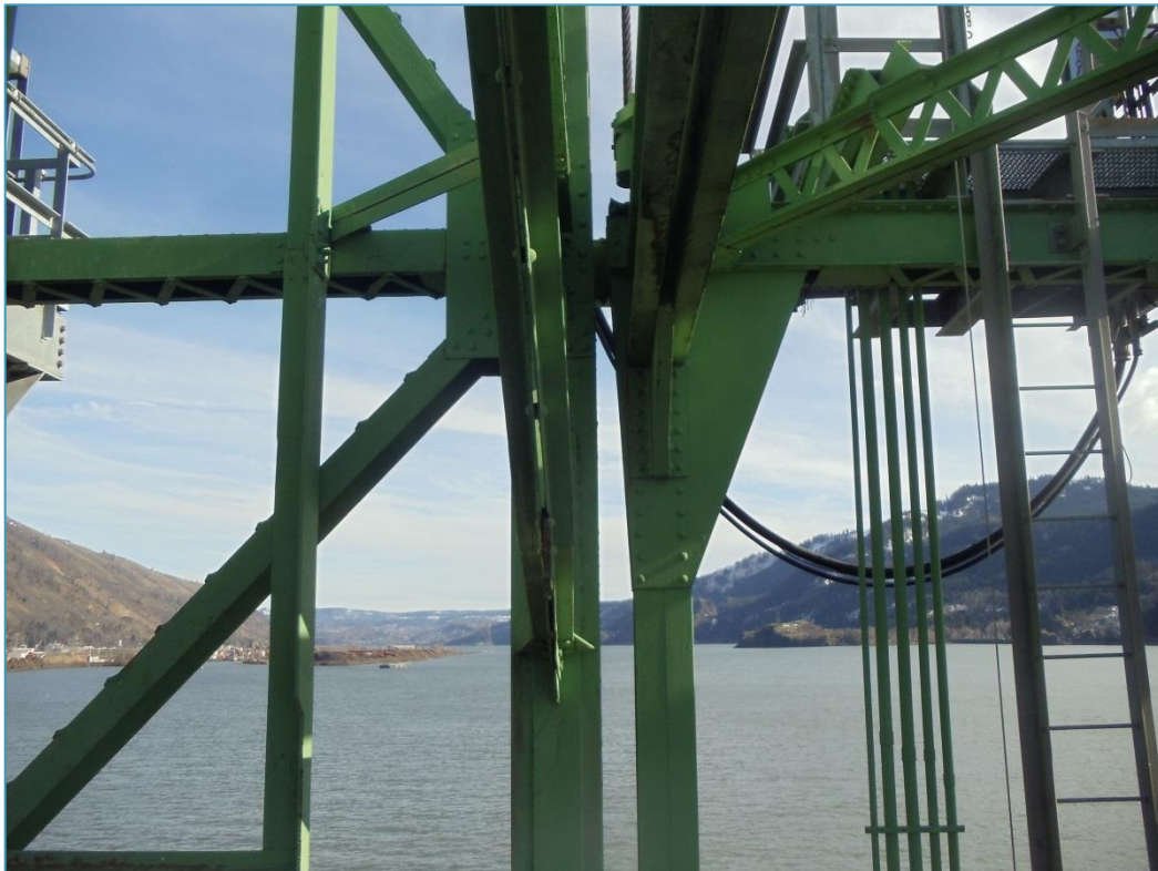
Alignment of eastern half (NB lane) of portal bracing.
