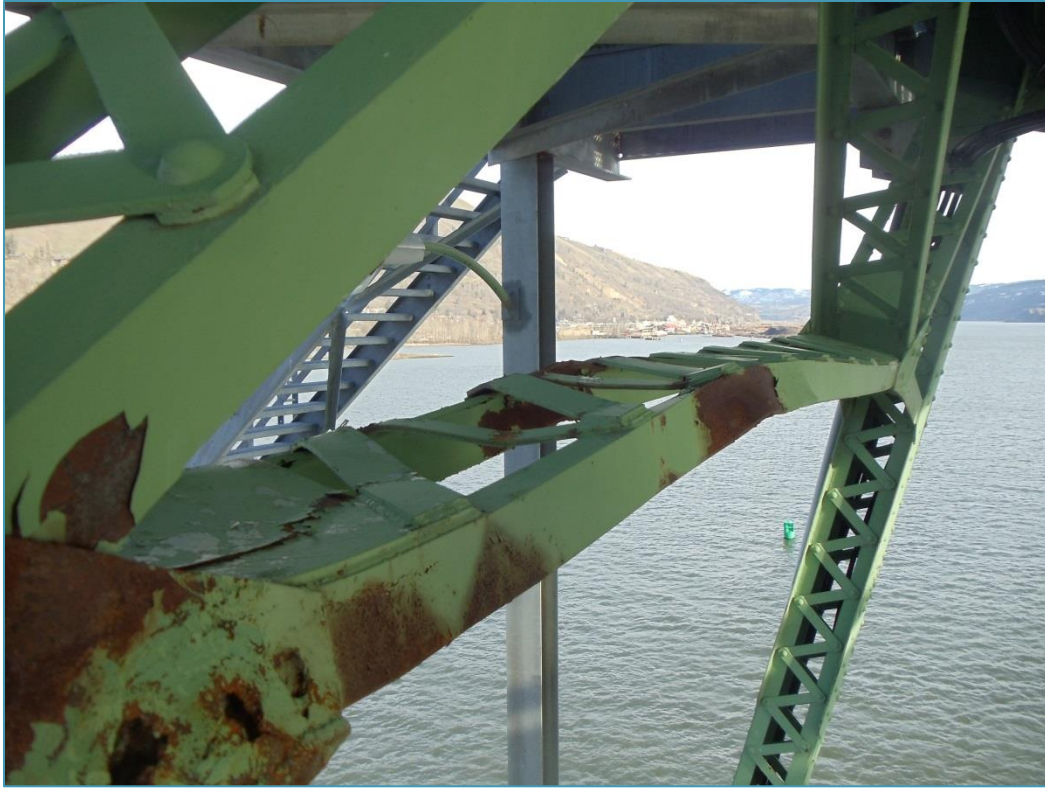
Horizontal strut at northernmost portal (back face of tower).
