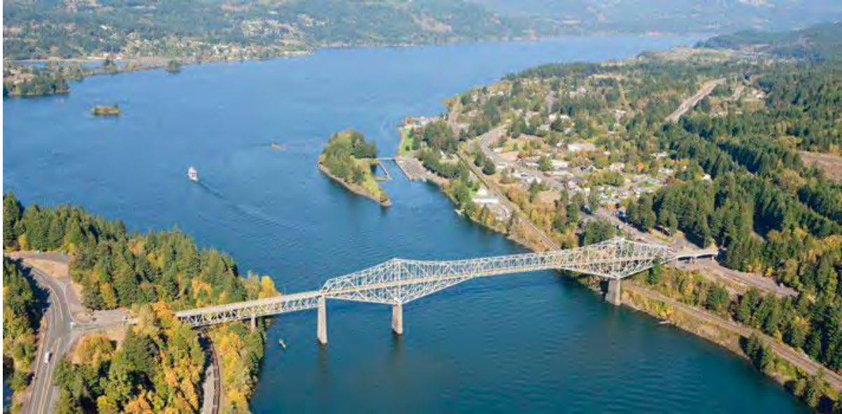
Photo Source: Hood River County
