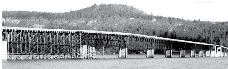
The Hood River Interstate Bridge was originally built in 1924, and essentially rebuilt in 1937 when the liftspan was added to accommodate heightened water levels created by Bonneville Dam. The Port of Hood River purchased the bridge in 1950, and has been responsible for maintenance and improvements for six decades.
