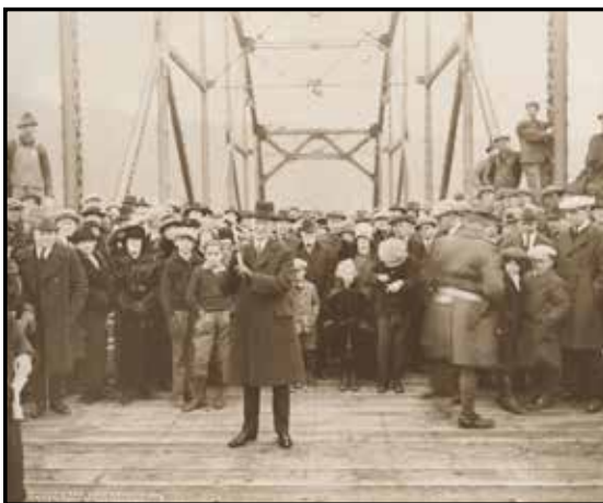
Leslie Butler driving the last spike in the wooden bridge deck December 6, 1924.
