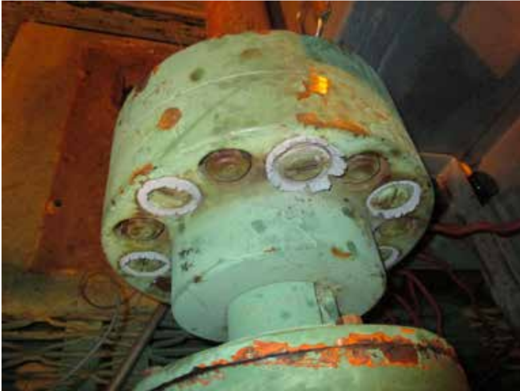
Photo 25. C1-SE. General View. The elastomeric inserts for the coupling bolts are deteriorated. The bolts and inserts are bound and could not be removed.
