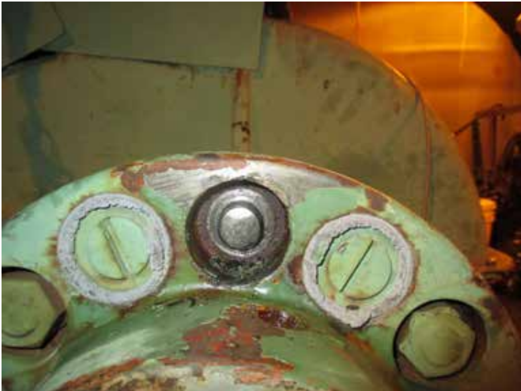
Photo 25. C1-SE. General View. The elastomeric inserts for the coupling bolts are deteriorated. The bolts and inserts are bound and could not be removed.
