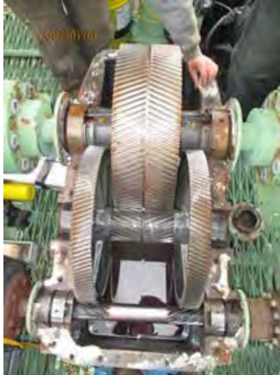
Photo 1. North Primary Reducer. General view of reducer with the top half of the reducer housing removed. The high speed end of the reducer is at the bottom of the photo.
