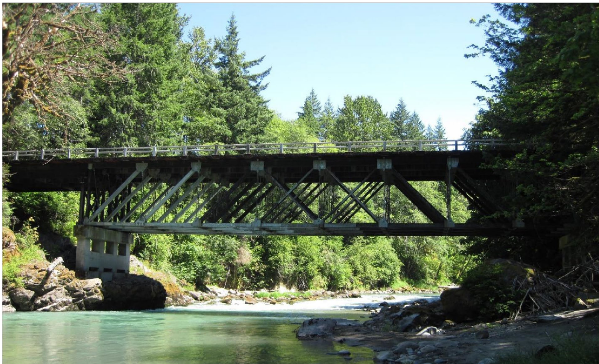
Huffaker Forest Service Bridge, Randall, WA – Live-load Test and Load Rating
