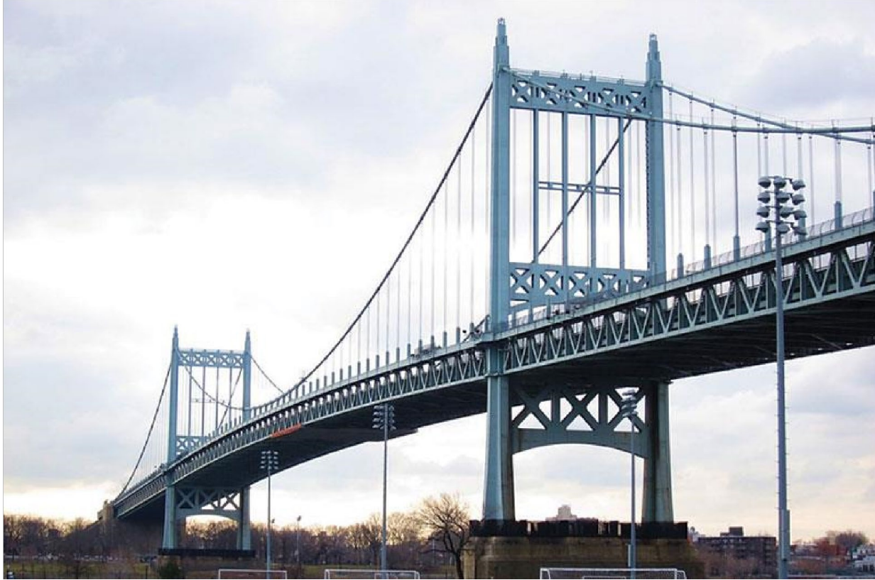
RFK Bridge Bronx, NY – Instrumentation and fatigue monitoring
