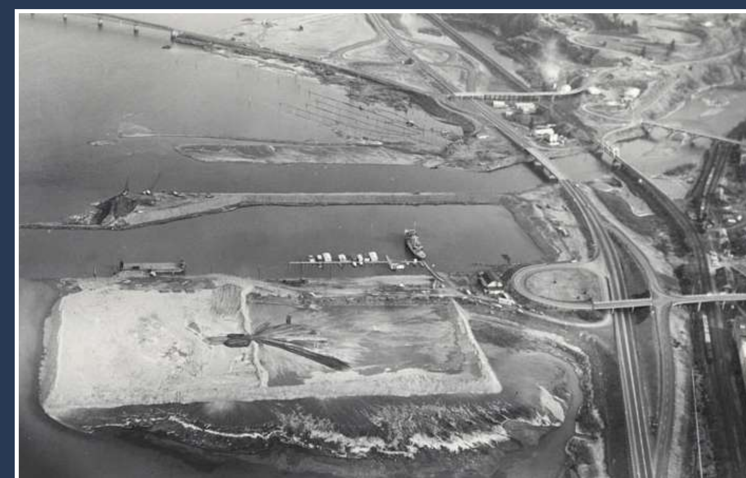
The construction of I-84 in the 1960s created a vast amounts of fill allowing for creation of Nichols Basin (seen here) and subsequent fill in the area at the top of photo which would become the Hood River Marina.
