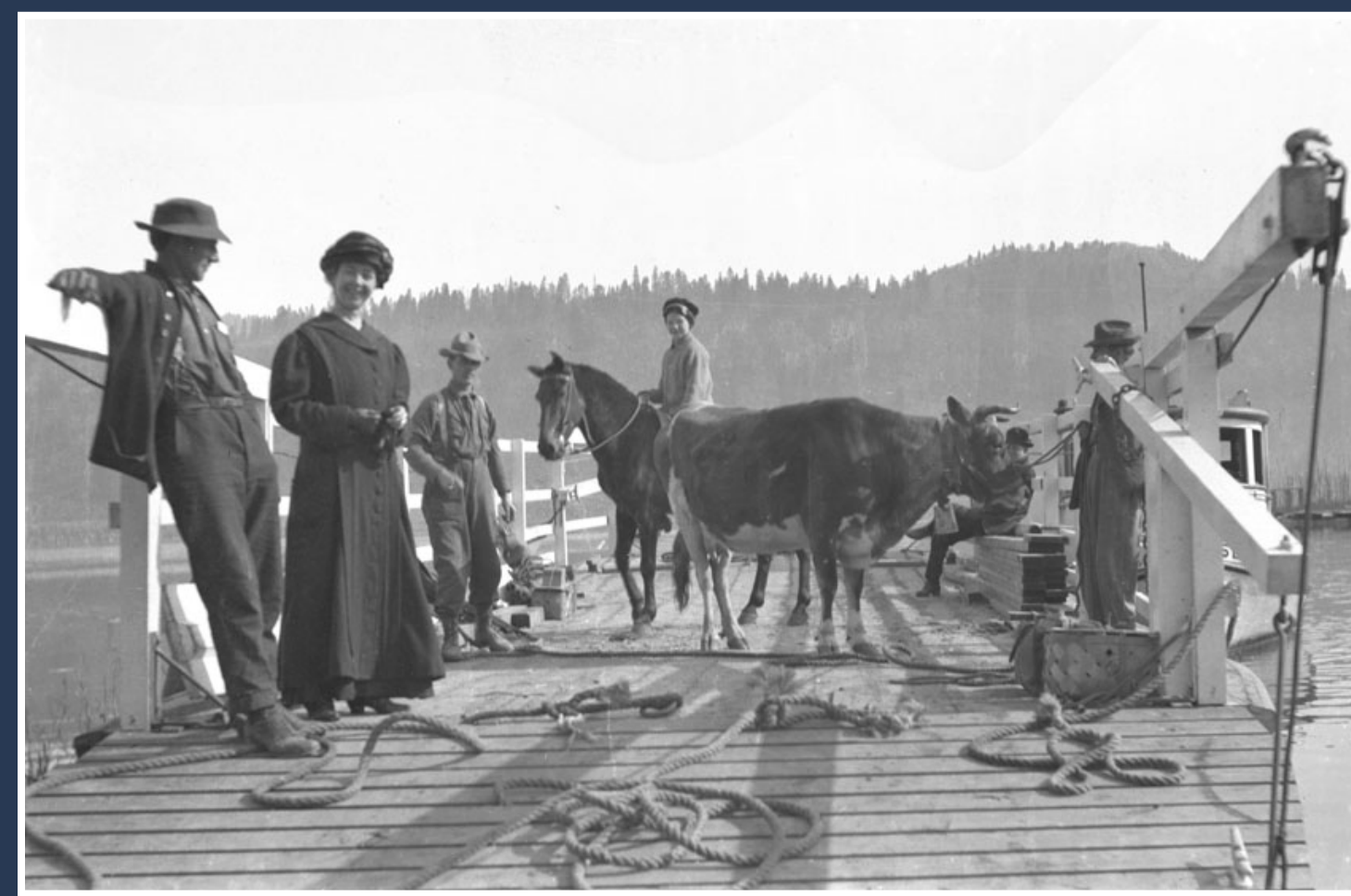
Prior to Bridge construction, locals, visitors and cows! crossed the Columbia on one of a number of ferry services.
