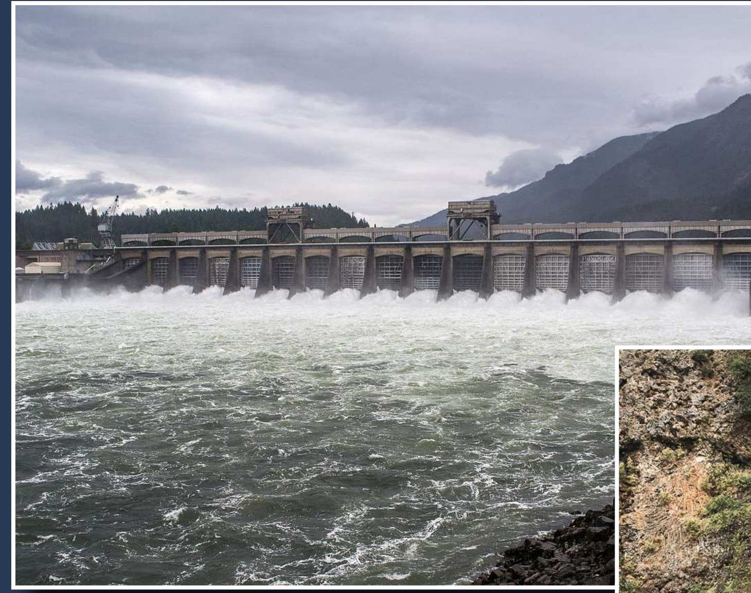
Bonneville Dams set the stage for power production and better navigation in 1938 and created the Bonneville Pool.
