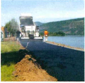
Crews pave a section of the existing waterfront path just west of the Event Site
