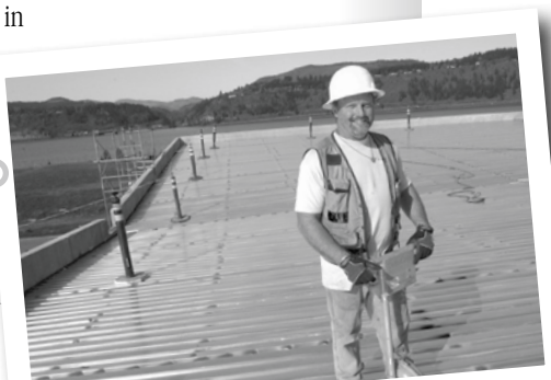
Halyard building roof decking installed
