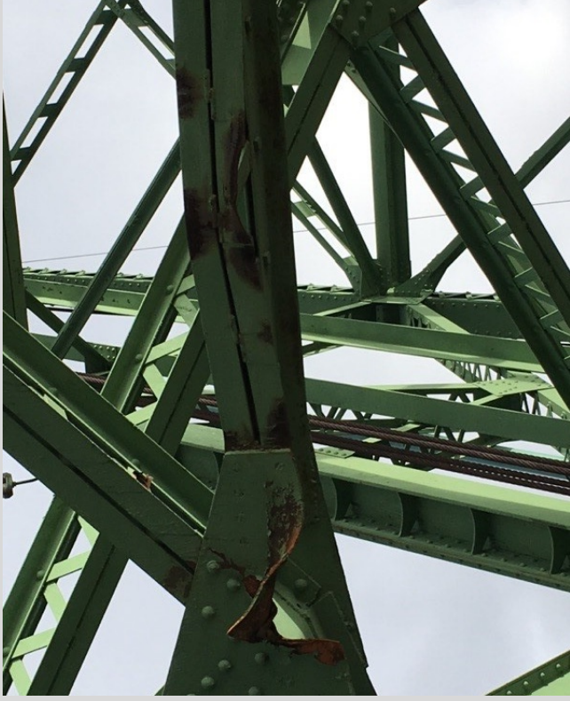
2019 Portal Truss Repair
