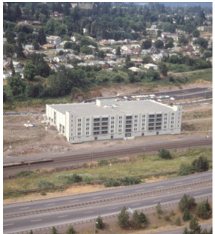
The Waucoma Center was transformed from a 50-year old cold storage plant was transformed into a modern telecommunications center.
