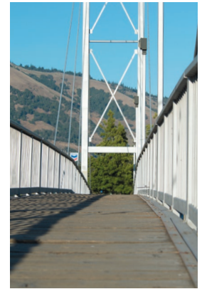
Pedestrian Bridge over the Hood River will receive a new deck and new lighting in 2022
