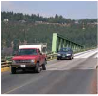
Cars exit the south end of the Bridge
