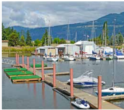
South Dock at the Marina
