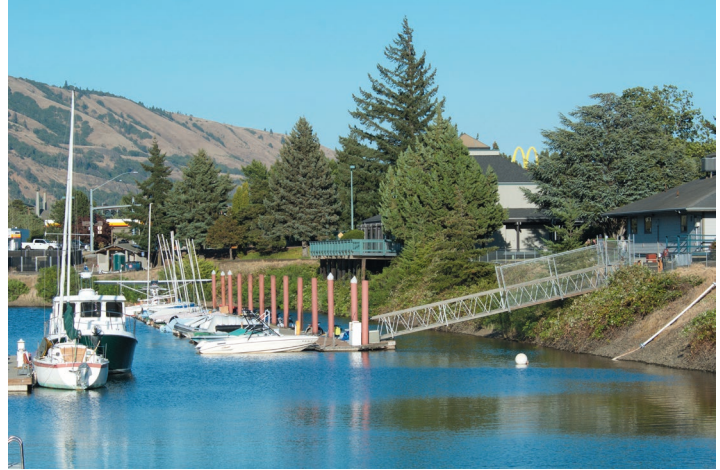
The South Basin Dock will be upgraded and expanded in 2024-25
