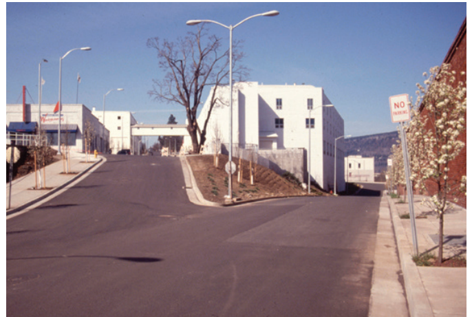
The late 1980's and early 1990s saw a dramatic transformation of the Columbia/IndustrialWasco Street areas.
