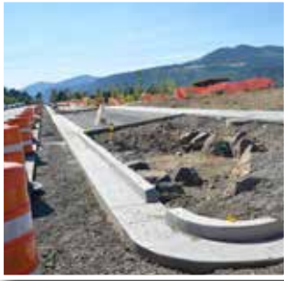
Parking improvements underway during the summer of 2013
