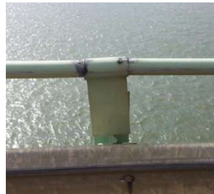
Figure 2. Span 16, P9 bent upper WT connection for pipe rail.
