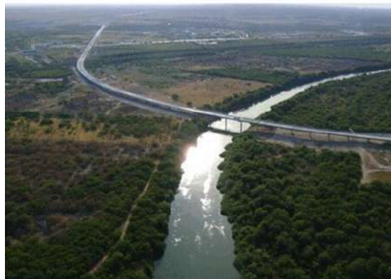
Anzalduas International Bridge McAllen, Texas - Reynosa, Tamaulipas (The U.S. is shown on the right.)
